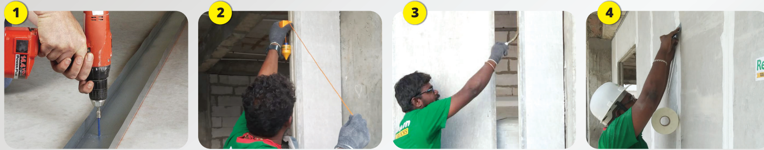
1 Fix Ceiling and Floor Channels
